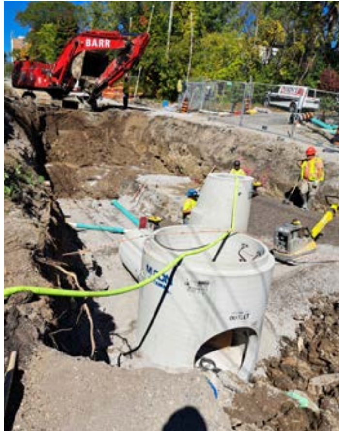
Photo: Sanitary sewers and watermain installation.
