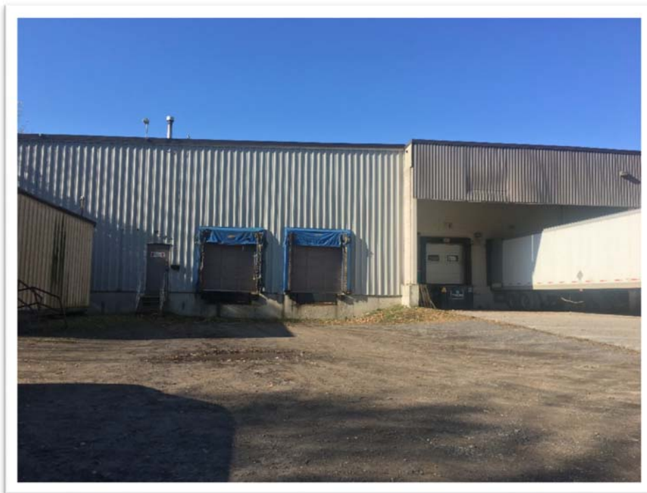
665 Dundas Street East – shipping/receiving loading area, view looking west.
