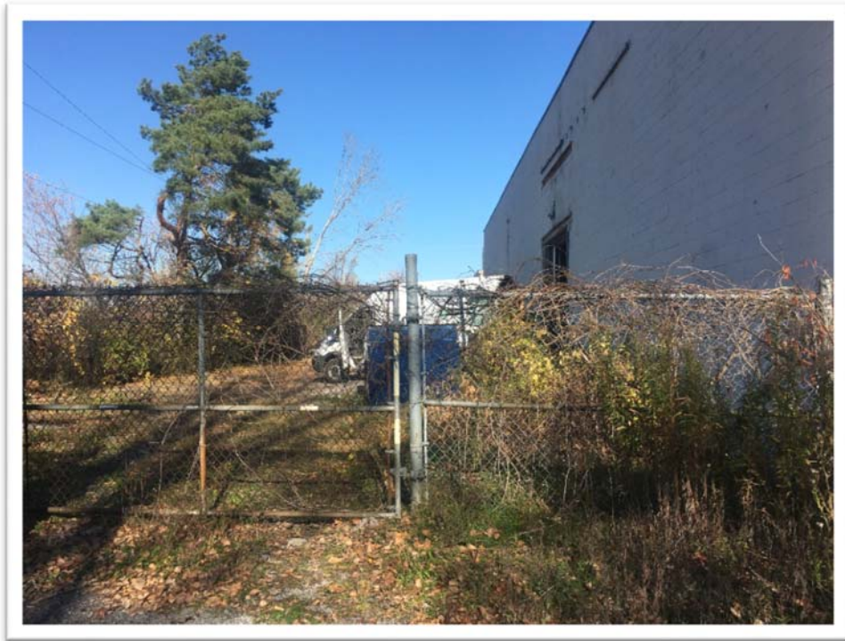
665 Dundas Street East – side yard, view looking north.
