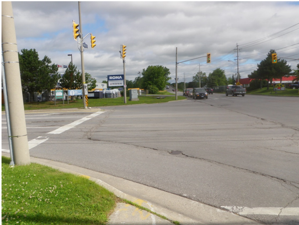
Plate 2: Looking north from the intersection of Bell Boulevard showing modern commercial/industrial properties and lanes narrowing to two lanes as approaching the 401 overpass
