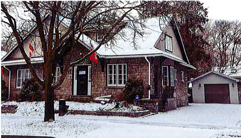
Example of a dwelling with a second unit in Belleville, ON
