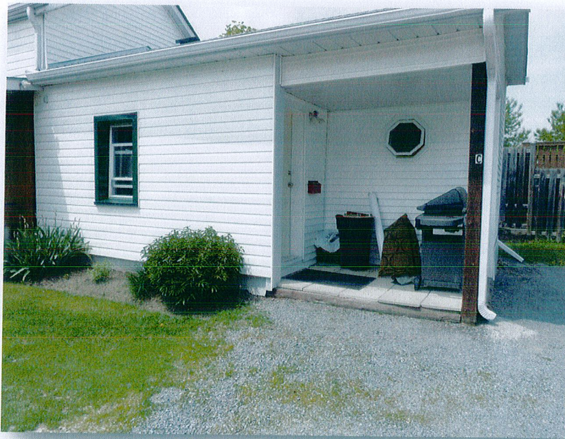
View from rear parking area (looking at Unit #2 entrance).
