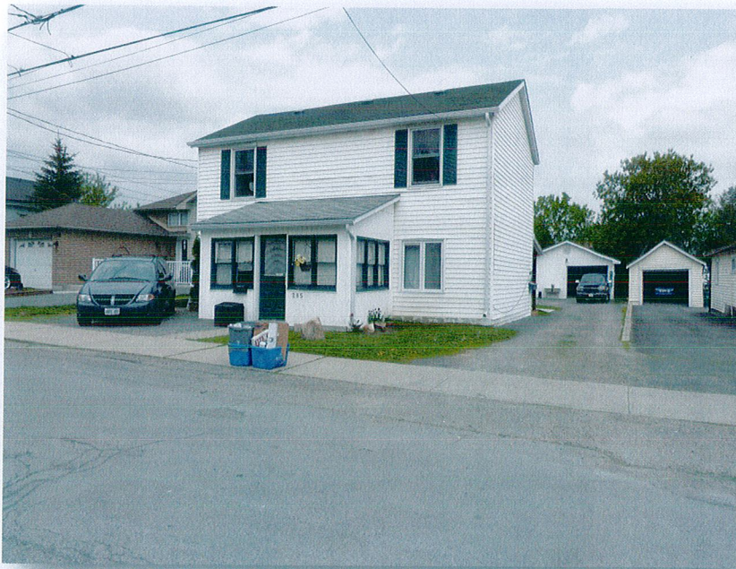
View from William Street (looking east).
