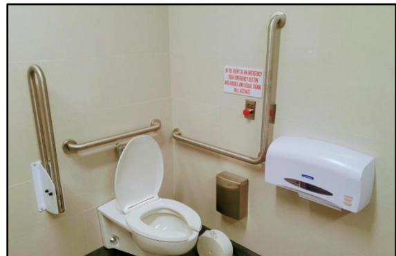
Photo Five: A fully renovated washroom with accessible features such as grab bars, toilet and toilet paper height placement, and an audible and visual emergency push button.
