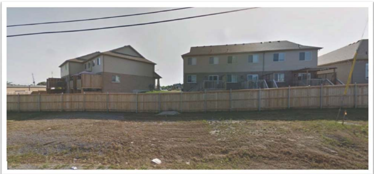
Townhouses across Street
