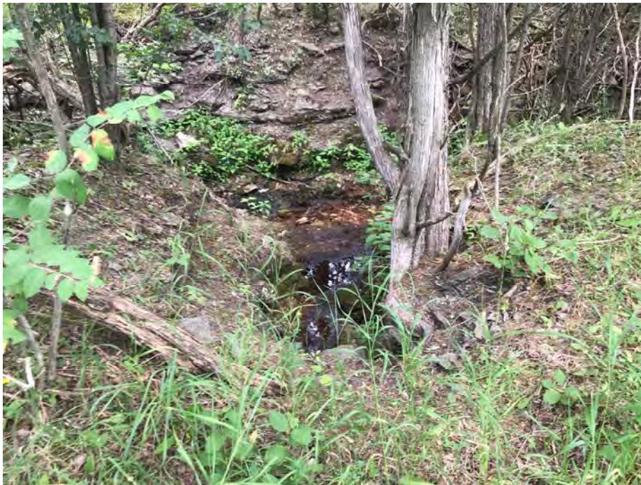
Photograph 6. July 11, 2019. Outlet of PSW unit to excavated channel, looking north.
