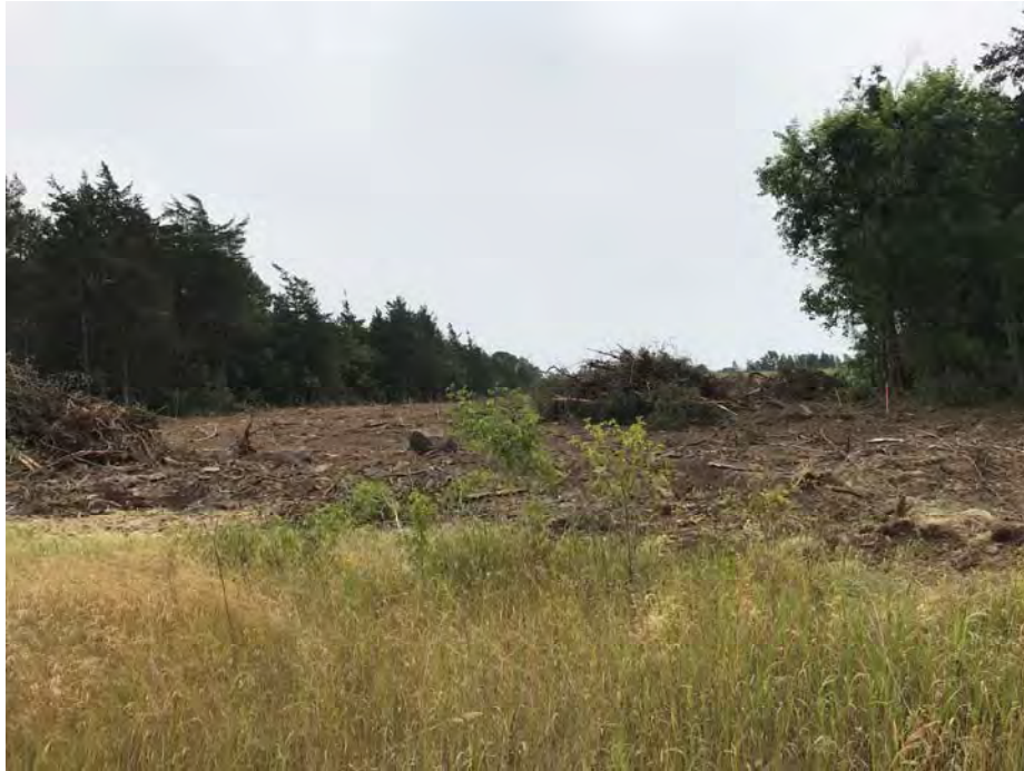
Photograph 9. July 11, 2019. Recently cleared area south of the northeast meadow, looking south.
