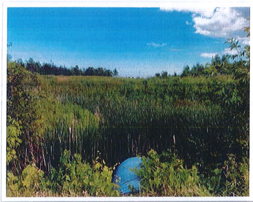
Lot 4 – view from Enterprise Drive looking south, culvert bottom-centre.
