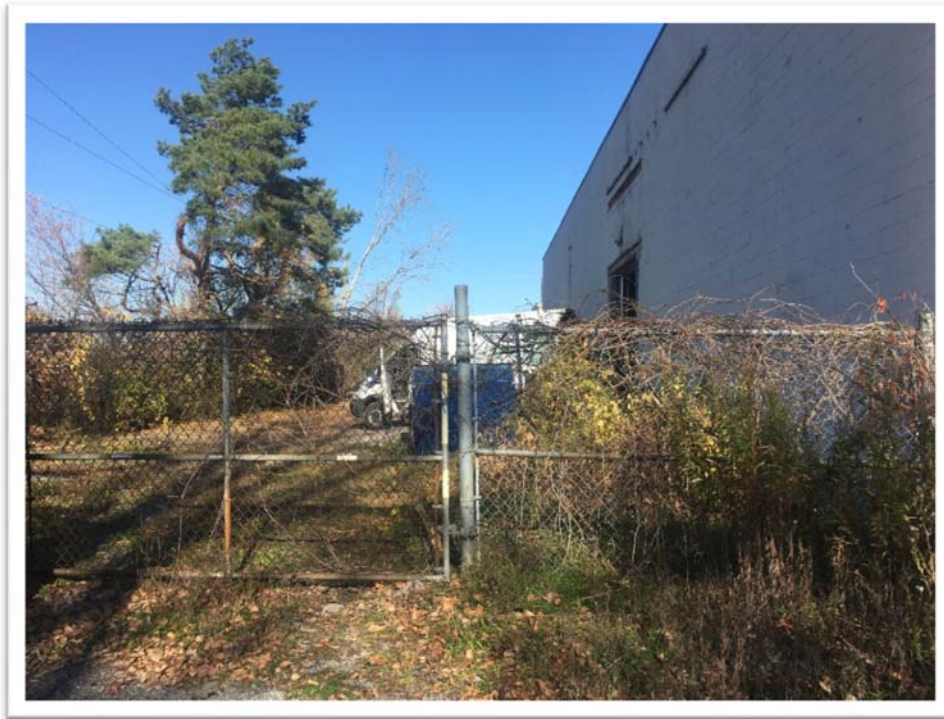
665 Dundas Street East – side yard, view looking north.
