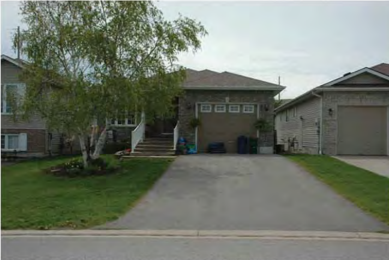
View looking west from Moira Lea Court (#17 Moira Lea Court pictured)
