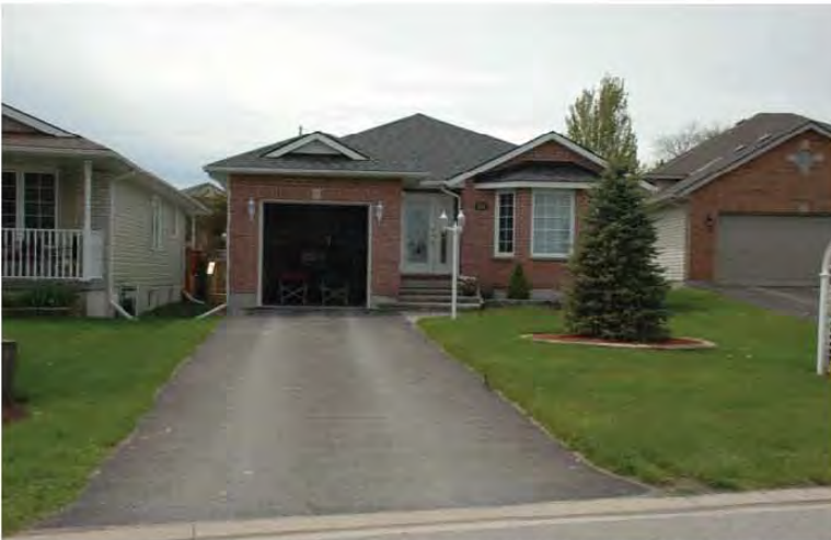
View looking west from Moira Lea Court (#21 Moira Lea Court pictured)
