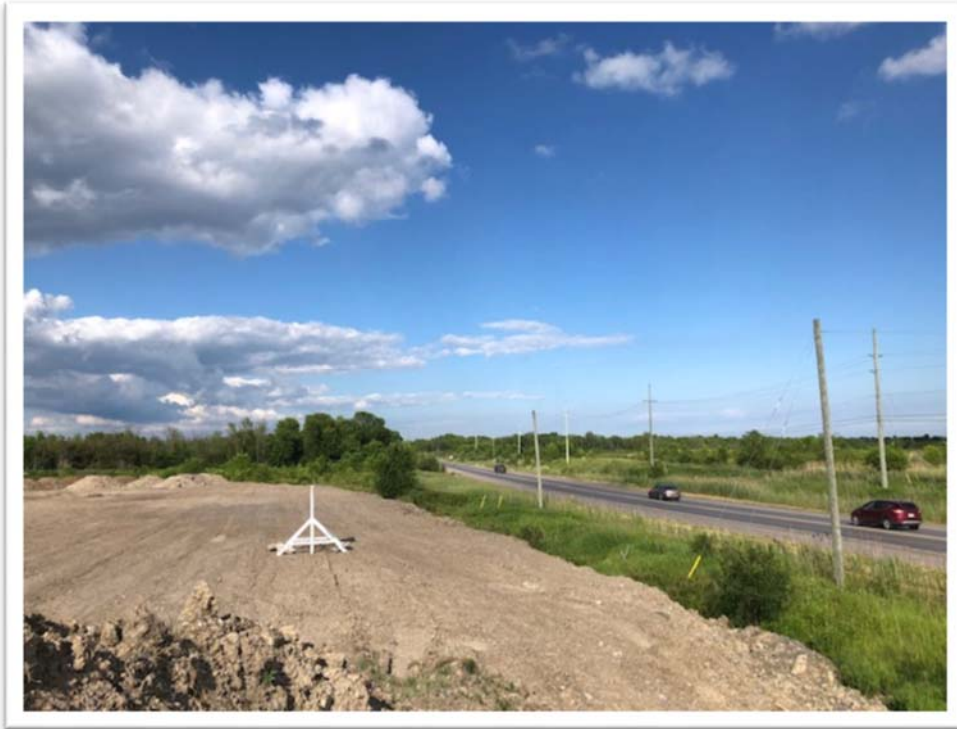
Lot 1 – view looking east along Bell Boulevard streetscape (right to centre).
