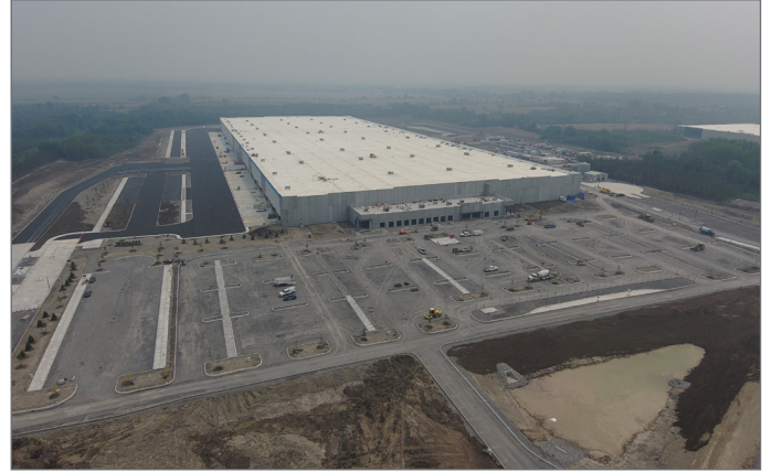
Photos showing the construction phases of the project.
