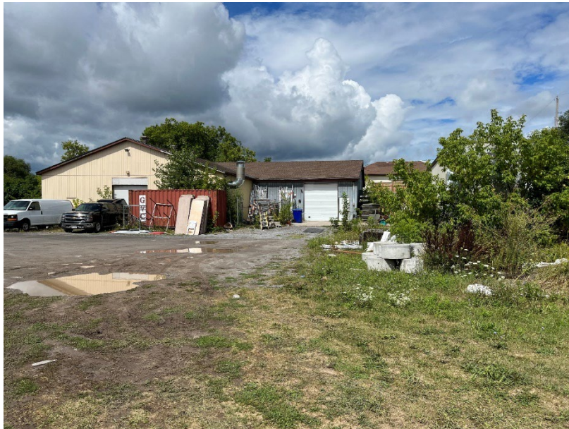
Photo 5: South side and rear of commercial building on subject property
