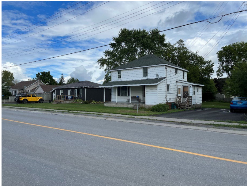
Photo 7: Adjacent house to north on Cannifton Road North
