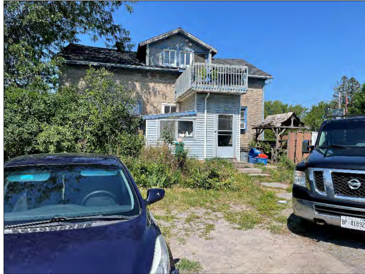
Back of residential house at west portion of 84 Cannifton Road N property. Photo is taken facing west.
