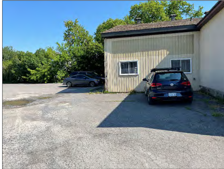
Side View of west side of main building at 84 Cannifton Road N. Picture taken facing north from west side of Site.
